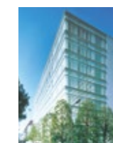
Nov. 2001– Current JICPA Building (Chiyoda-ku, Tokyo)
